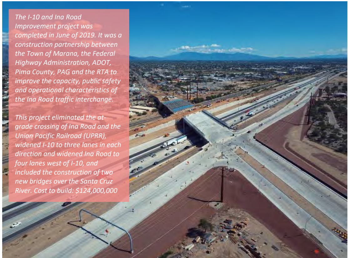
Ina Road construction. Source: Psomas
