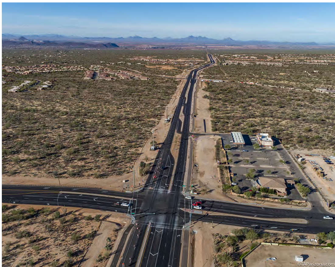
View west of the Tangerine Corridor from Thornydale Road. Source: Town of Marana
