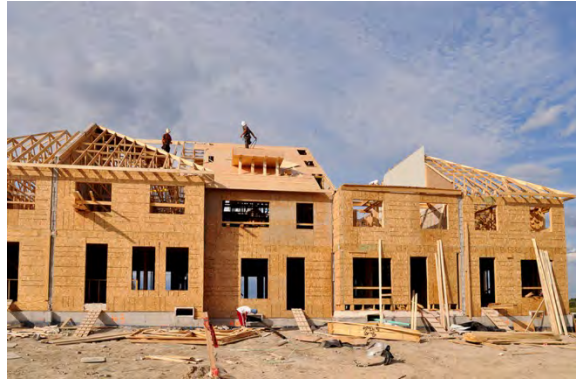
Construction in Marana. Source: Town of Marana
