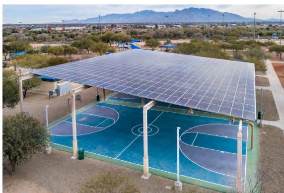
Solar Panels in Crossroads at Silverbell District Park Source: SOLON Corporation
