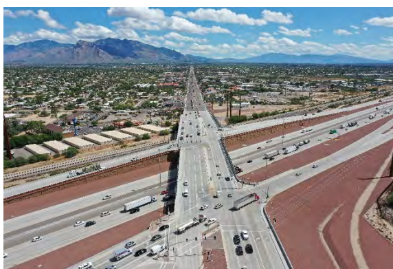
Aerial view of the Ina Road Corridor, east of the Ina Road Interchange on Interstate 10.
